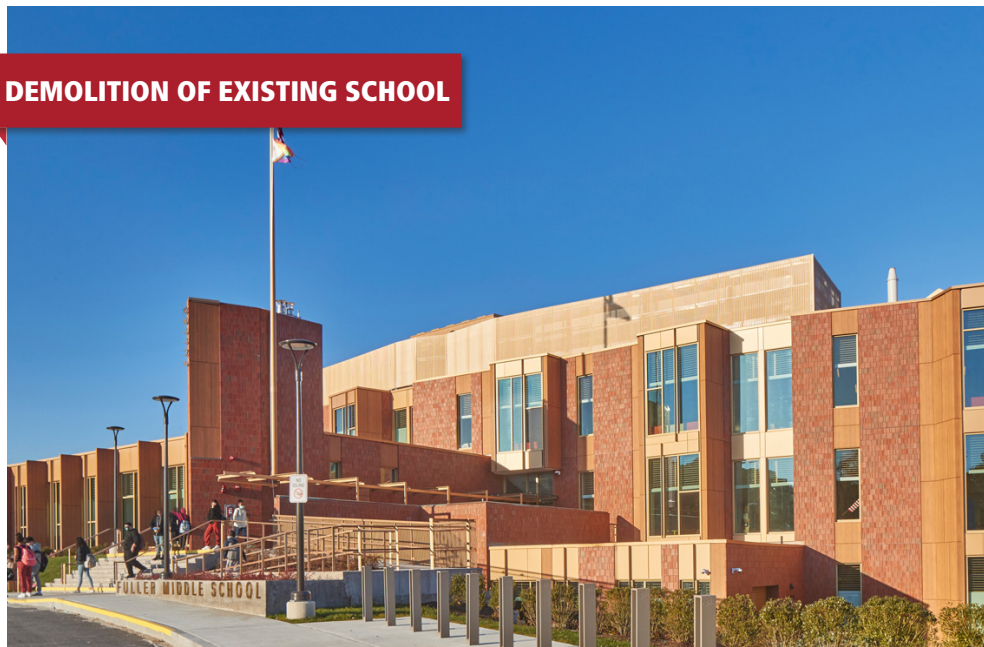
City of Framingham Fuller Middle School
