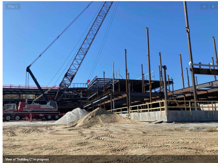
View of "Building C" in progress
