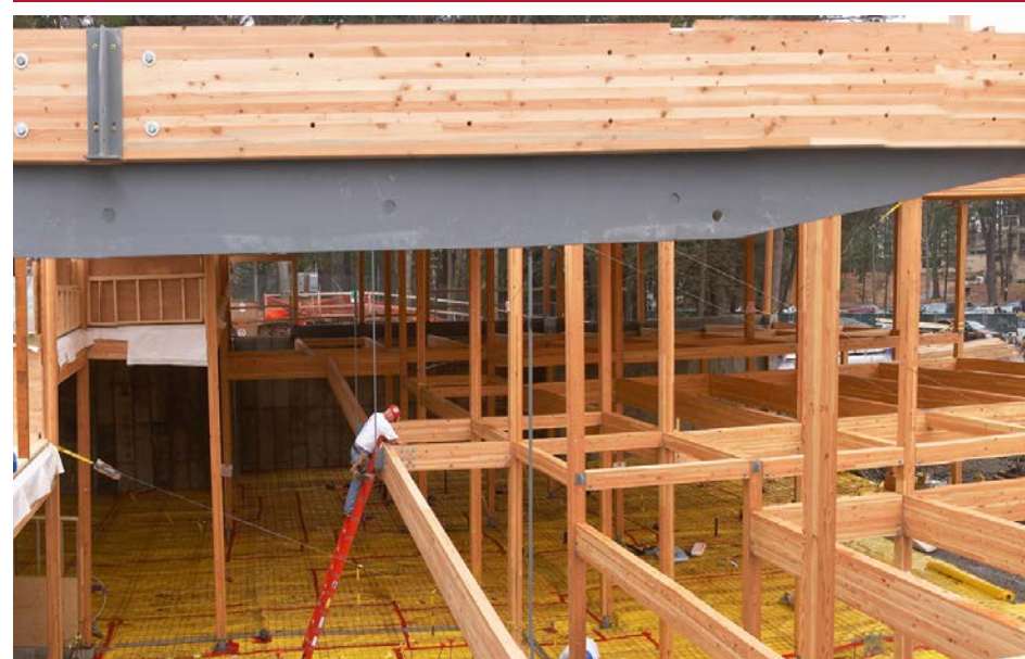
Mass Timber Framing
